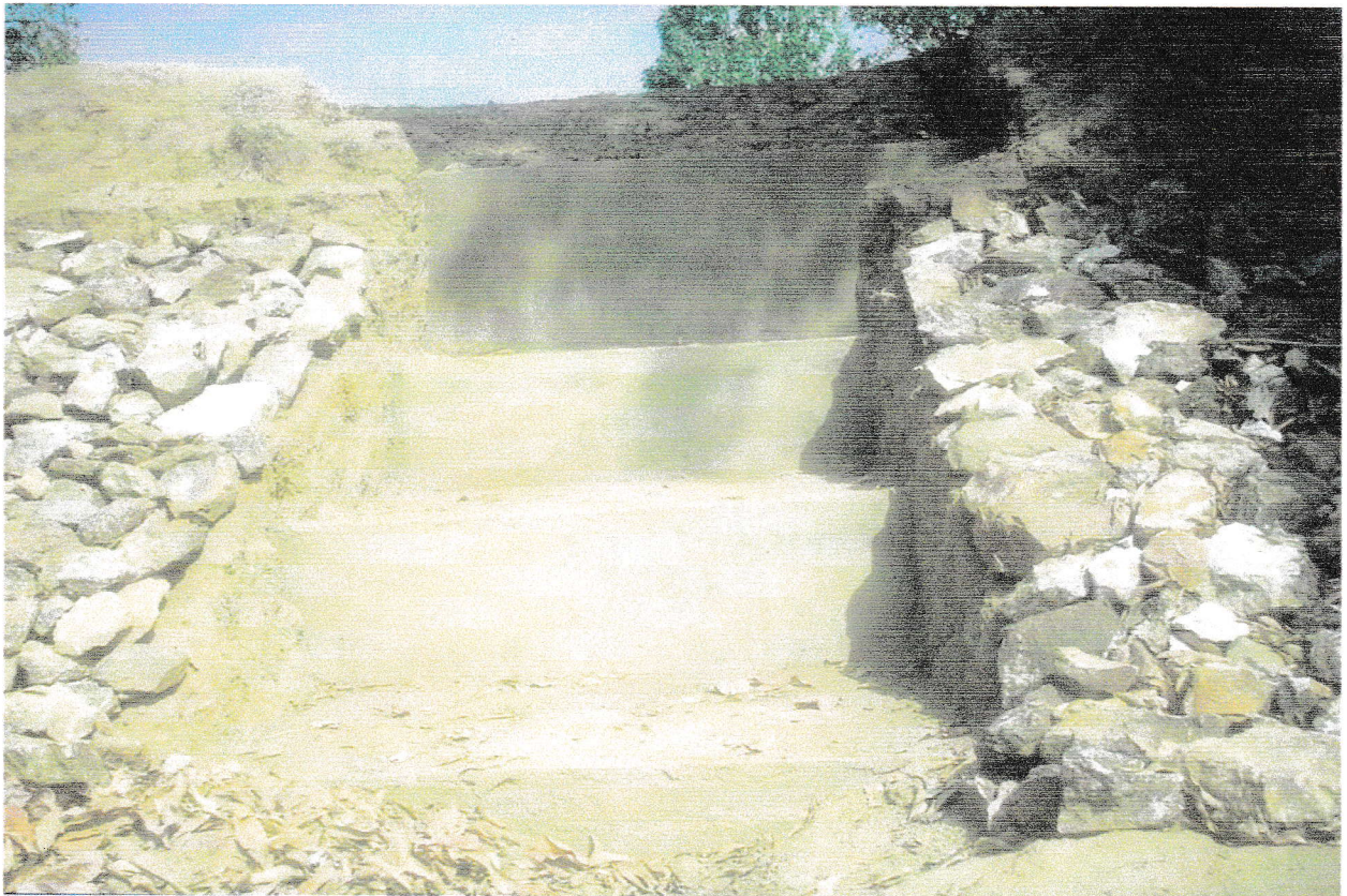
New constructed Plug Type Head Regulator at R. D. 260 Mtr.
