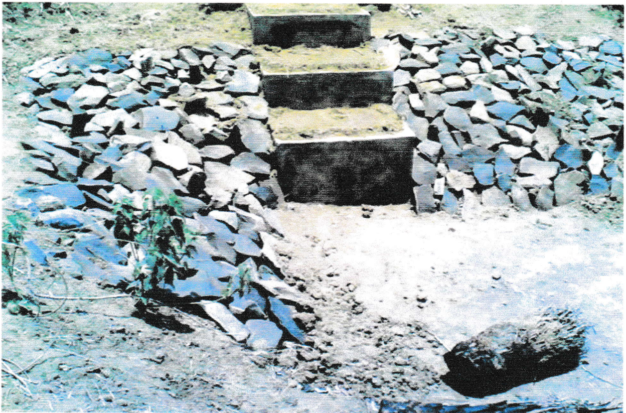
New constructed Head Regulator at R. D. 595 Mtr.
