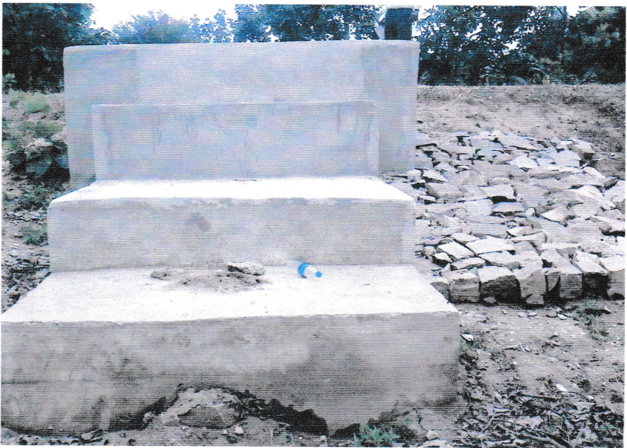
Newly constructed Plug Type H. R. at R. D. 10 Mtr. with D. R. Pitching.
