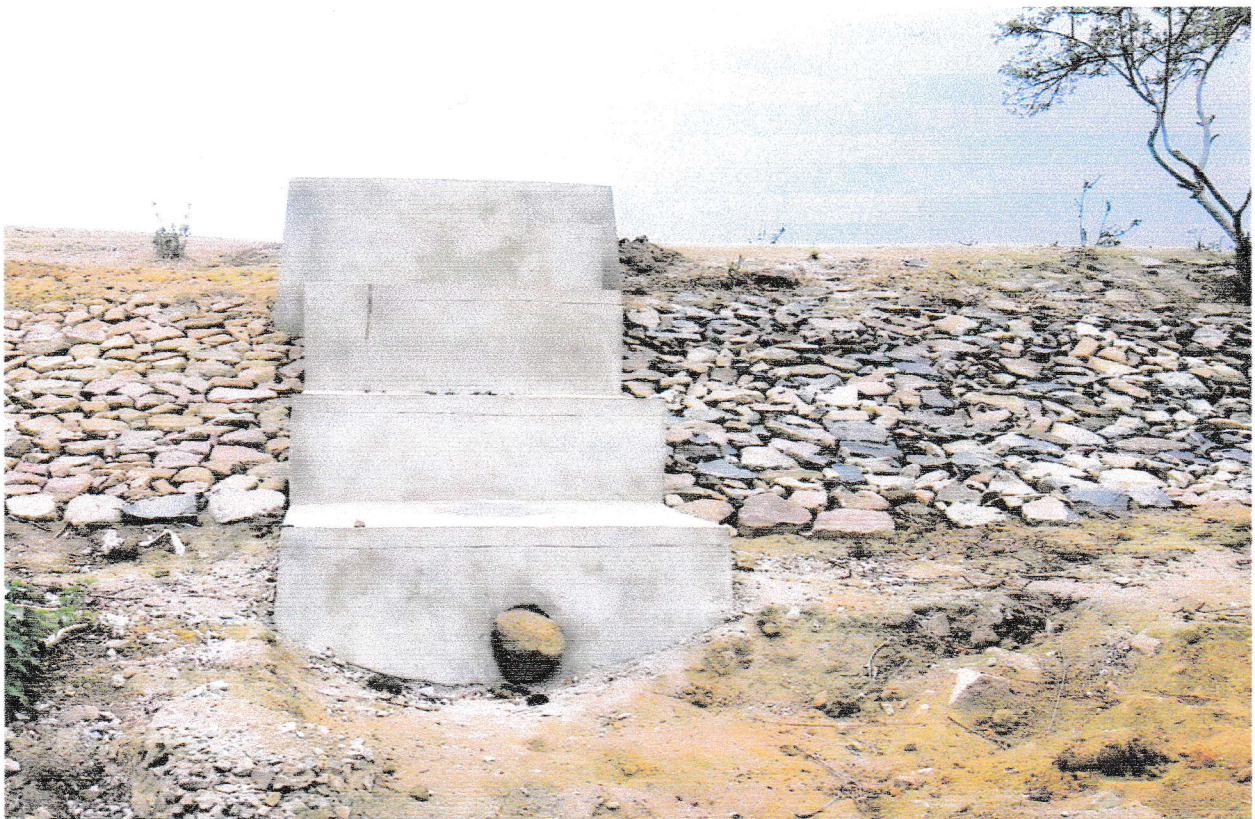
Newly constructed Plug Type H. R. at R.D. 140 Mtr. with D. R. Pitching.
